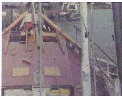
The Coach-Roof and Decking taking shape
